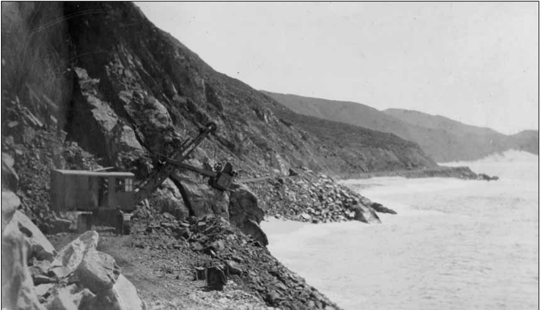
Construction of coast highway, looking east from Point Mugu c1924. Dewey C. Alderson Album, MVC
